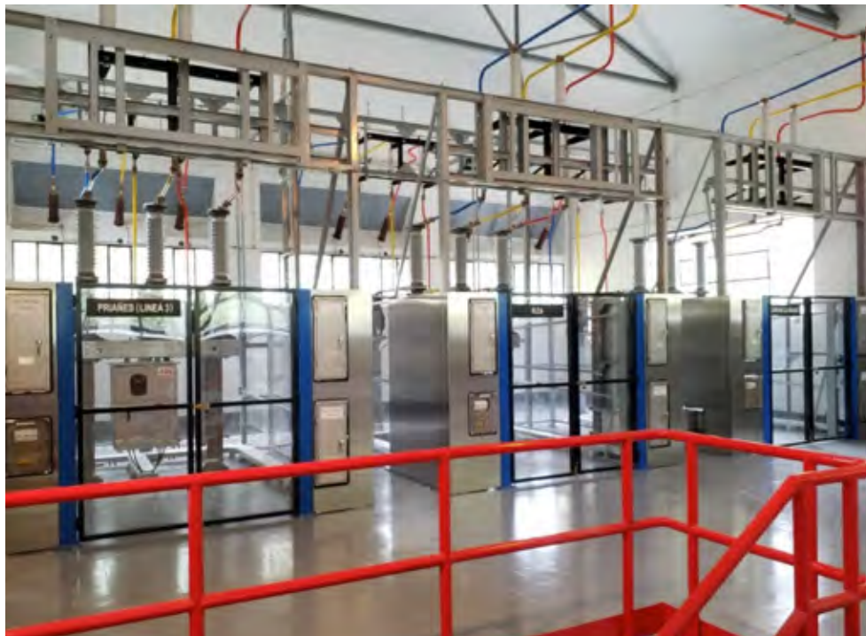
View of the finished works
