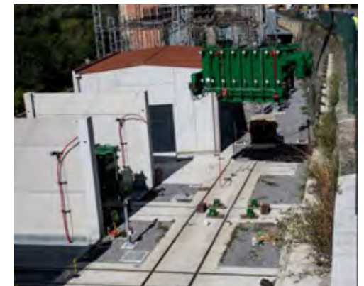
Installation of the new transformer
