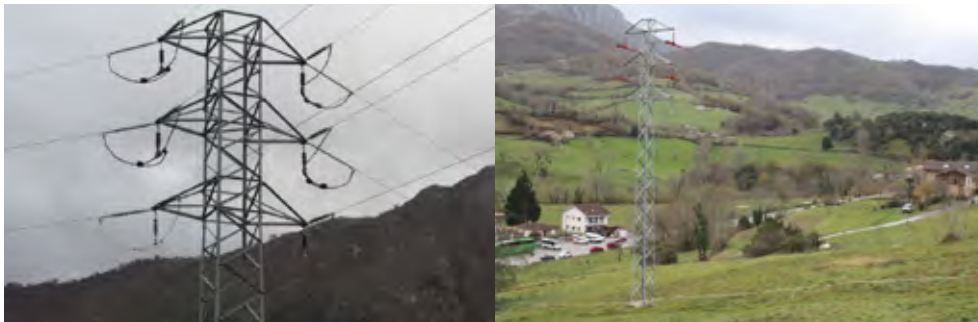
Support with changed insulation
